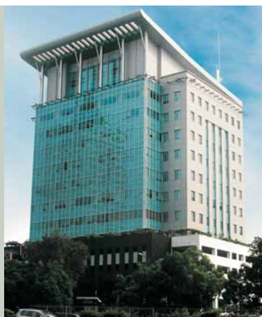
I.K.P.T. Office Building
